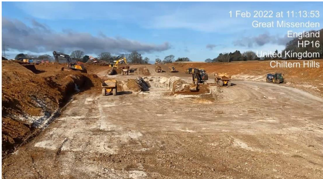
Excavations at the South Heath cutting – 1 st Feb 2022
