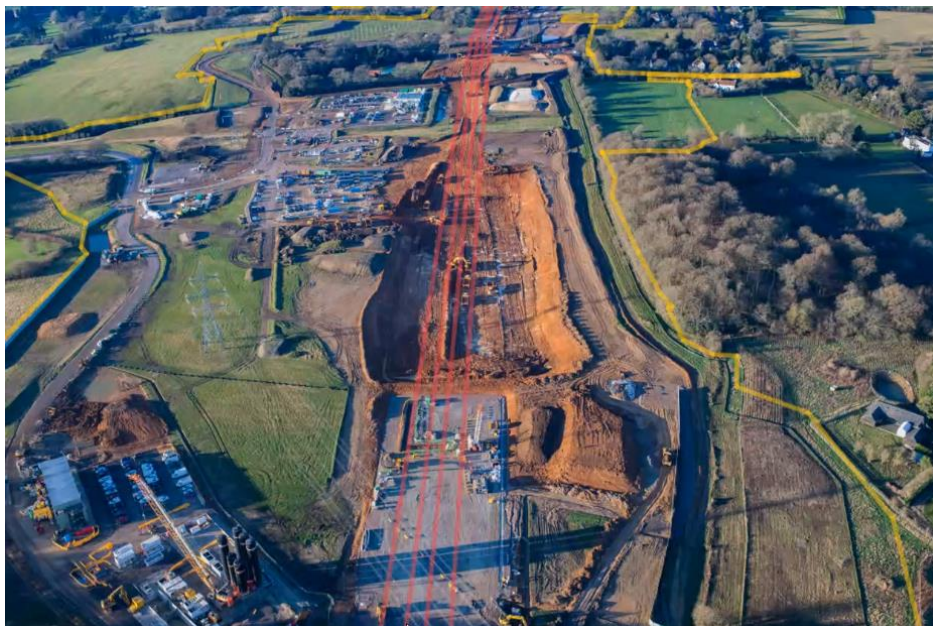
Excavation at South Heath, showing the area in the foreground in which 'barrettes' will be sunk and the start of the cuttings heading north
